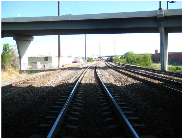
Figure 23 Denver, South Park & Pacific (5DV.6243.8) Looking North from beneath the US-6 Overpass
