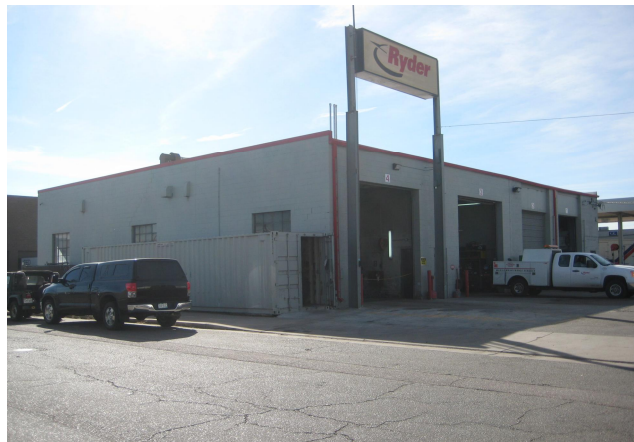
Figure 13 535 Alcott Street (5DV.11268)
